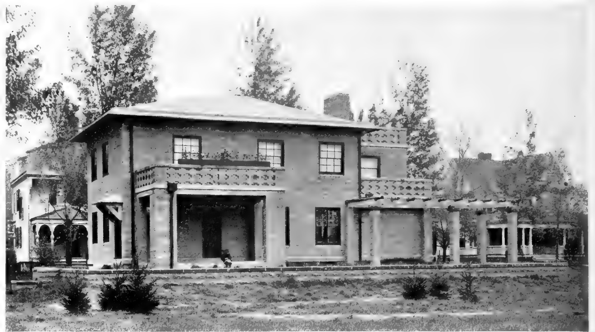
12—House of Mr. W. J. Steel, at New Dorp, Staten Island, is Constructed with Hollow Block Walls and Reinforced Concrete Roof and Floors
